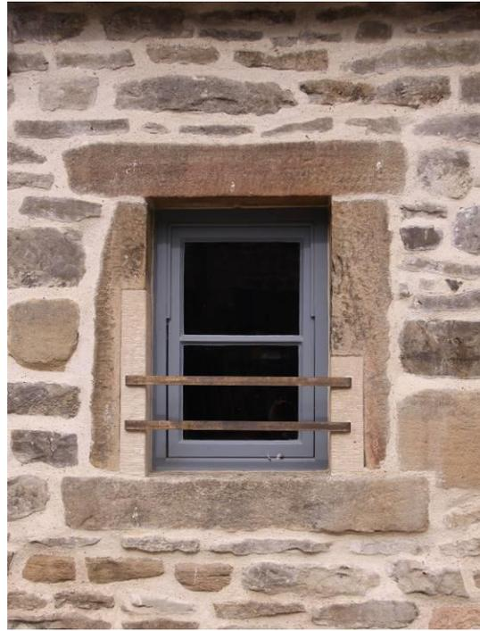
A like-for-like replacement of an historic window, including stonework repairs and new ironwork, based on evidence from the existing openings. (© Bench Architects)
