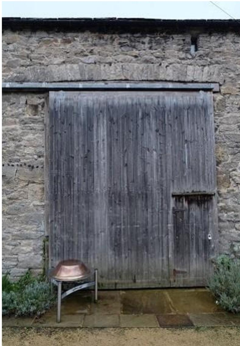
The 20<sup>th</sup> century sliding door on this threshing opening, although not part of the original building, has been retained and can be closed to cover the new glazed opening behind it. This maintains the agricultural feel of the converted barn and helps to tell part of the building's history.
